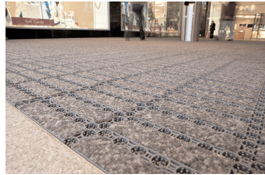
Plymouth's Drake Circus used Syncros' expertise to ensure the right matting was installed
